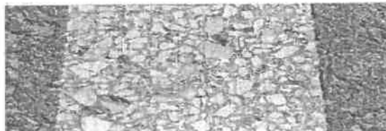
Figure 7. Photo of an asphalt cement concrete groove with a light corduroy pattern, made with properly spaced, gang-stacked cutting blades.
