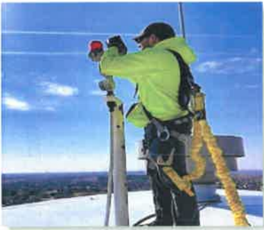
A Public Works employee replaces a warning light on top of the west water tower.
