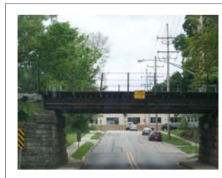
UPRR Rail Bridge on Pearl St. in DeKalb
